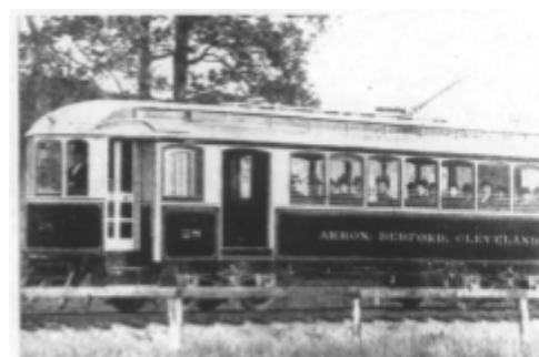
Figure - ABC interurban line, courtesy of the Olde Northfield Historical Center
